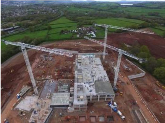
Following the erection of Tower Crane No 3 (three more to go!) the superstructure frame to the Diagnostic & Technical Block and the first ward areas have quite literally flown up. This part of the building is currently at Level 2, with columns in place to support Level 3.
